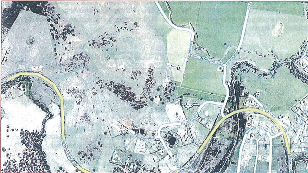
Figure 3 Aerial photograph of the site showing small lot development on adjacent land
